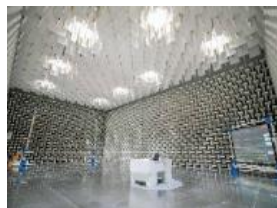
10m Anechoic Chamber
